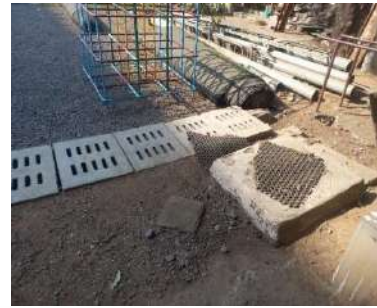
Underground rain water harvesting tank
