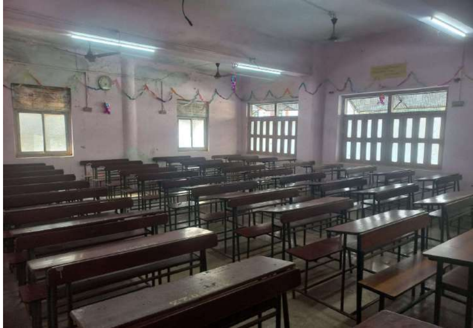
Class Room with proper cross ventilation and sufficient window
